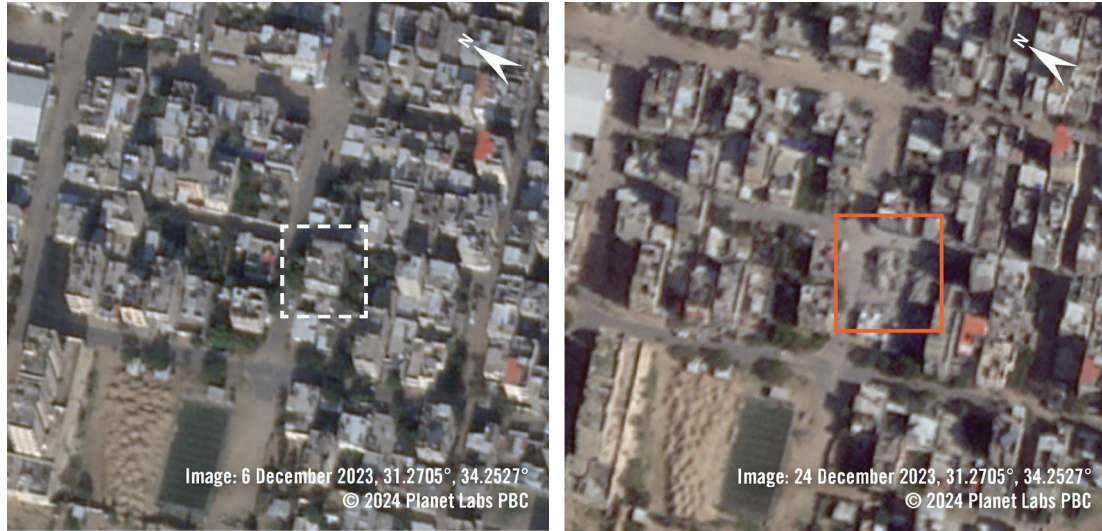
👁️ ↑ The satellite imagery from 6 December 2023 (on the left) shows the three-storey house of the Shehada family in Rafah. The satellite imagery from 24 December 2023 (on the right) shows the house destroyed, as highlighted by the orange box.
