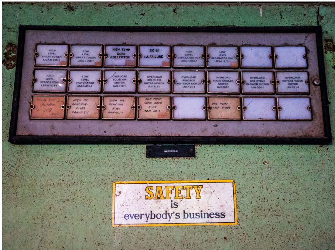
Control Room Details, Derelict Bhopal Processing Plant © Giles Clark 2014
